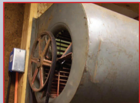
A low-speed squirrel cage blower motor
